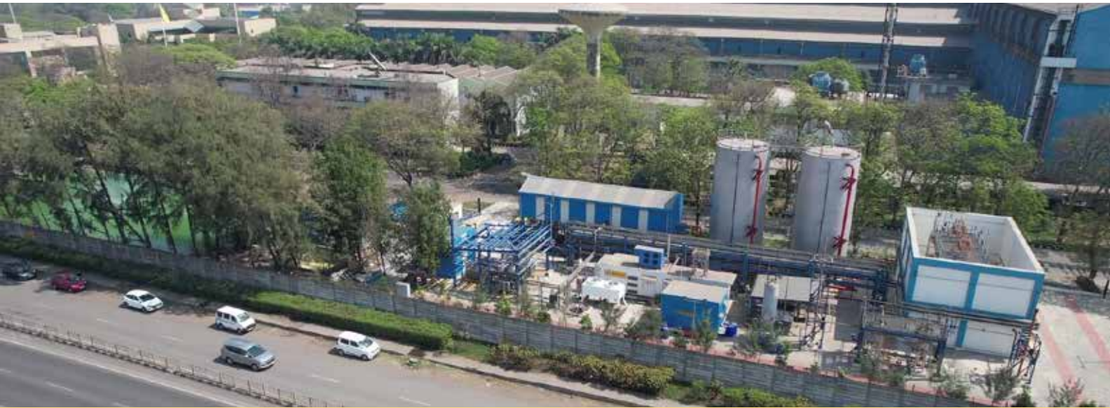
Green Hydrogen Plant at L&T's A. M. Naik Heavy Engineering Complex in Hazira, Gujarat
