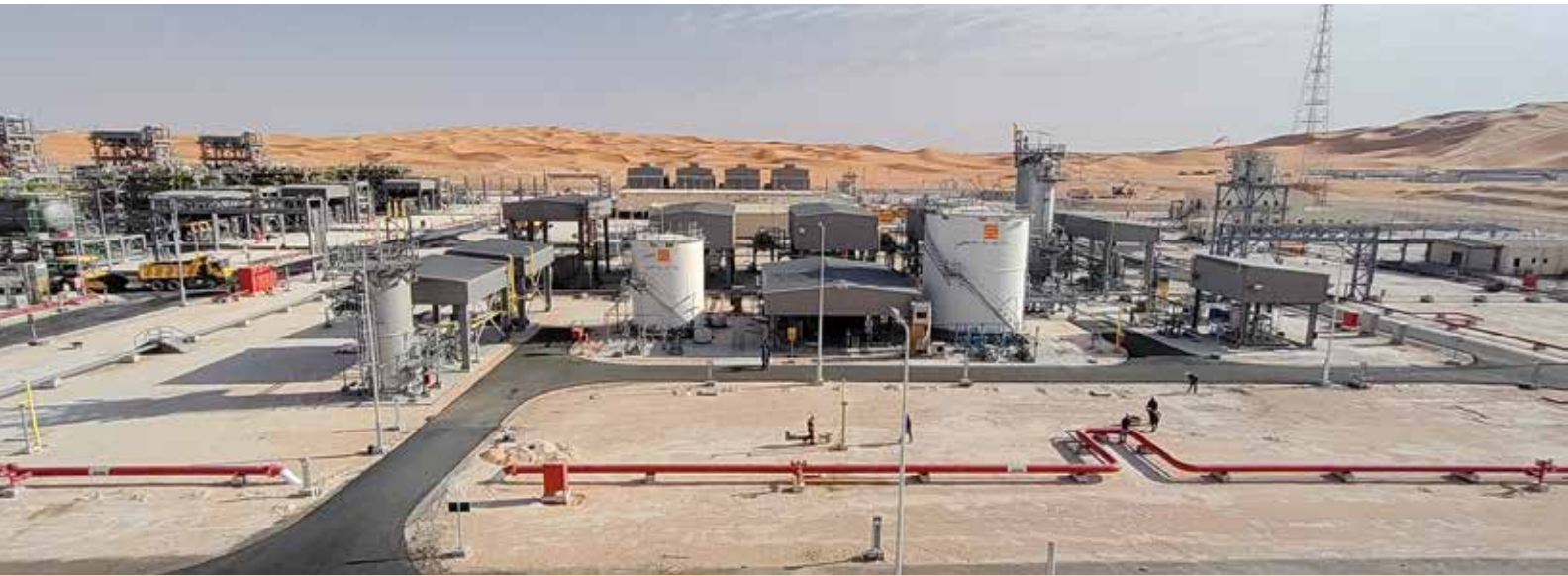
Central Processing Facilities for Sonatrach project, Algeria
